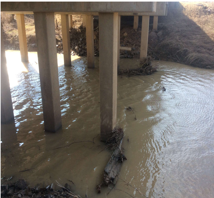
PHOTO 1 Description Channel - Spans 2-4 (small amount of debris)
