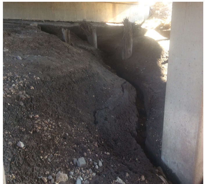
PHOTO 2 Description End slope near bent 6 abutment has erosion to channel bank.
