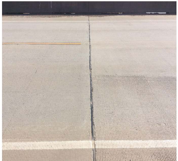
PHOTO 2 Description Joint - Bent 5 (losing adhesion)
