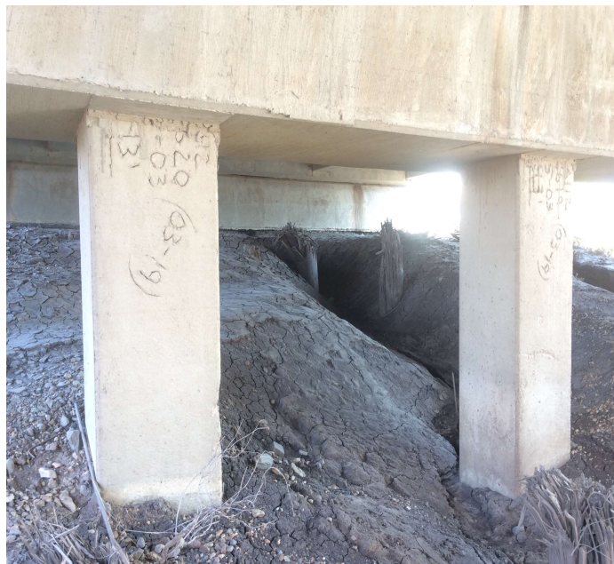
PHOTO 1 Description End slope - Span 5 (erosion)
