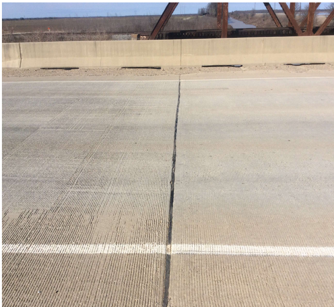
PHOTO 1 Description Joint - Bent 2 (losing adhesion)
