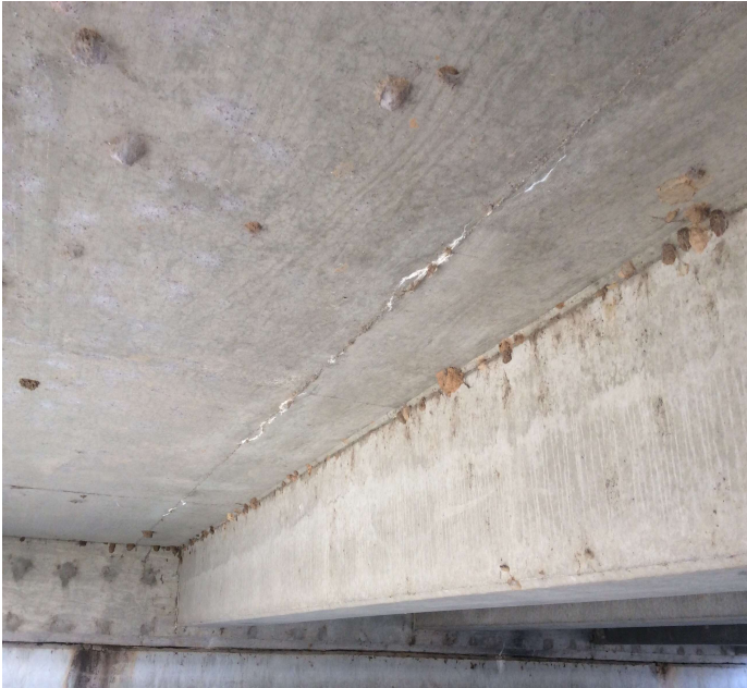
PHOTO 3 Description Soffit - Span 1 Bay 4 (efflorescence)
