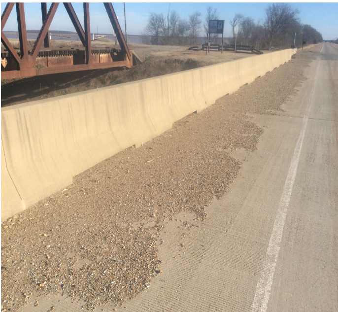
PHOTO 1 Description Left gutter line has gravel and dirt restricting storm water run off.
