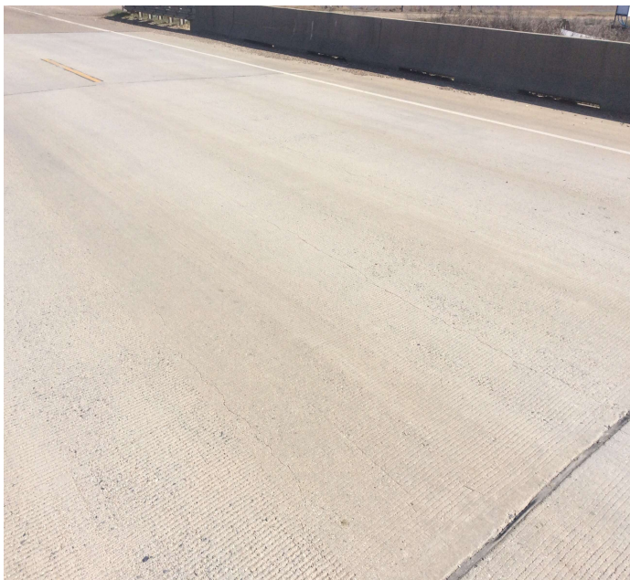
PHOTO 1 Description Deck - Span 4 (longitudinal cracking)
